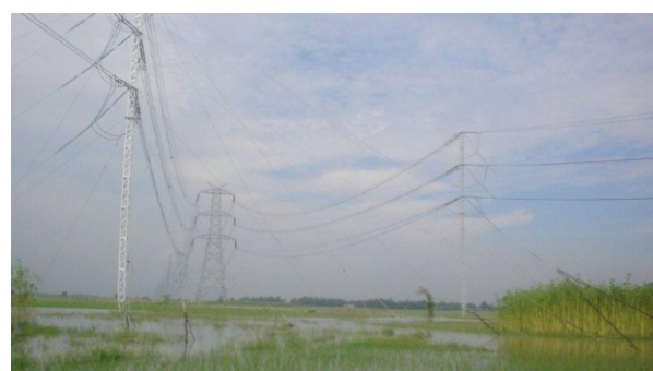
Emergency Restoration System deployed in Siliguri- Purnea line
