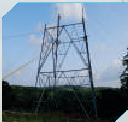
Tower Erection at 98/1 (Pkg-A)
