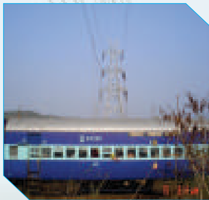
Stringing under progress at 41/0 – 42/0 (Railway X-ing) (Pkg-B)
