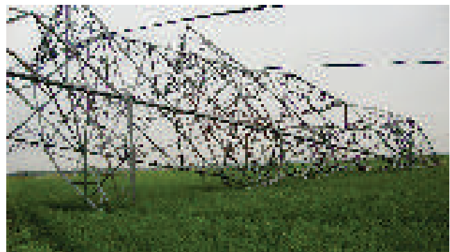
Tower Failures
